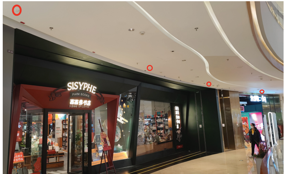
FIGURE 1. BLE beacons are deployed on the ceiling.
